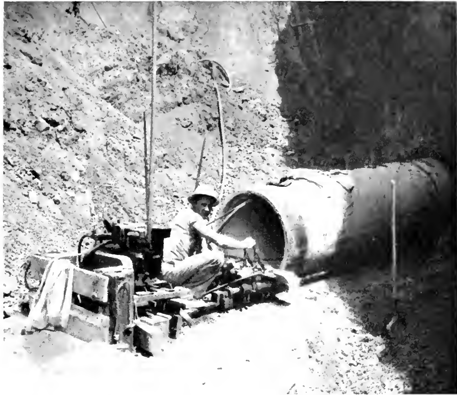
Jacking operation at Kellagg Hill
